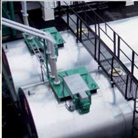
Horizontal Bitumen Tanks
