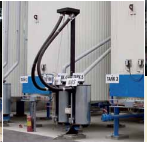
Bitumen Clean Fill System
